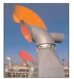
passive ventilation with heat recovery at BedZED
