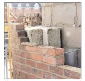
super-insulated masonry walls even out temperature differences in the buildings to negate the need for a conventional heating system
