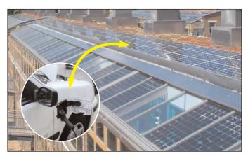
In order to avoid over sizing the CHP unit 1,138 photovoltaic cells have been installed at BedZED providing 109kW at peak output (the equivalent of enough electricity to power 40 electric cars to run 10,000 miles each a year. Photovoltaics are expensive to install compared with conventionally generated electricity this project demonstrates what can be done by using their three-fold functions of energy generation, solar shading and external cladding i.e. providing the "skin" of the building.
