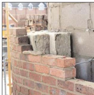
super-insulated masonry walls even out temperature differences in the buildings to negate the need for a conventional heating system
