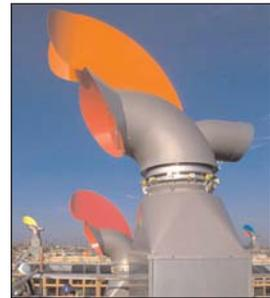
passive ventilation with heat recovery at BedZED
